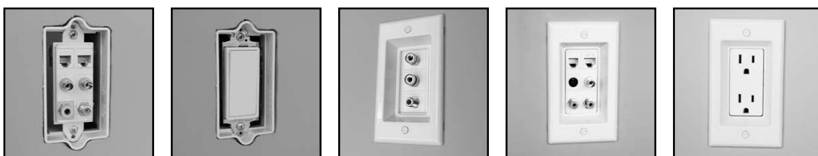
Typical finished installations
